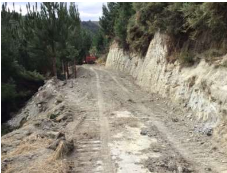
Photo 1: Track maintenance with excavator on Thompsons JV forest. Photo Josh Penn.
